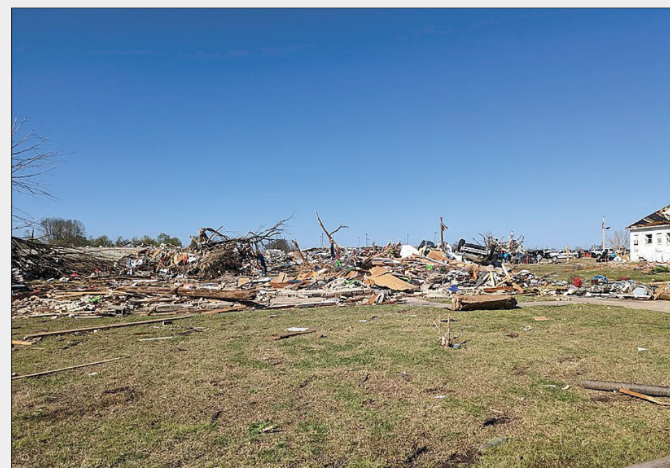
An image near Rolling Fork, Miss. one of the many devastations left by an EF-4 tornado that ripped through the South Mississippi Delta, Friday night, March 24. PHOTO COURTESY OF NOAA
